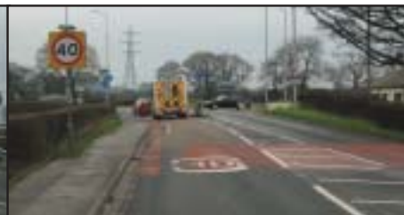
Fig 4 – Pedestrian / Cycle route sign obscuring roundabout signing.
